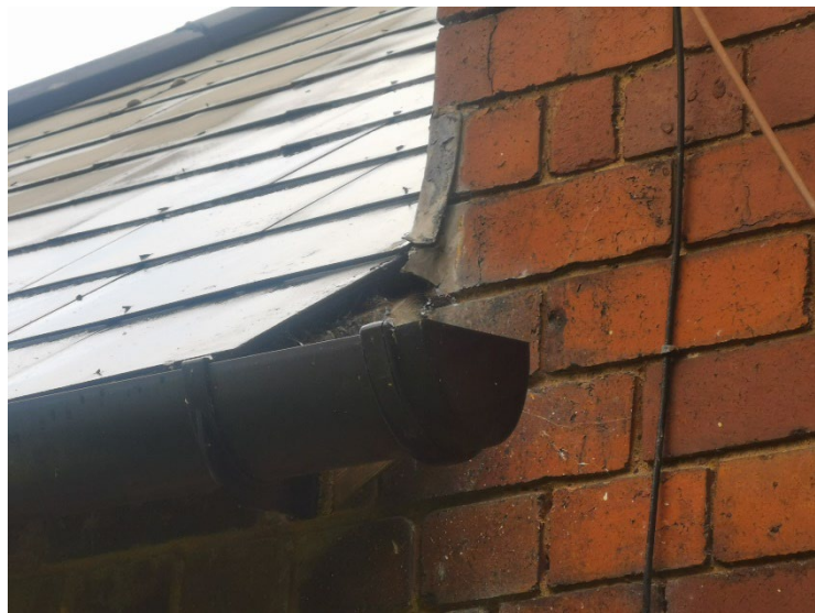
Building 11 – Gap under roof tile on southern face of the property
