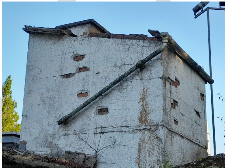
Building 12 – Crevices around exposed bricks and under roof tiles on office building
