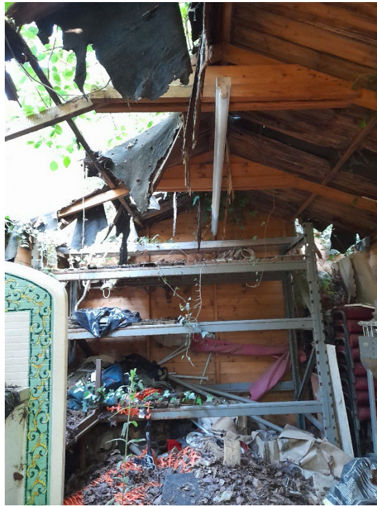
Building 13 – Sports pavilion shed with roof fallen through
