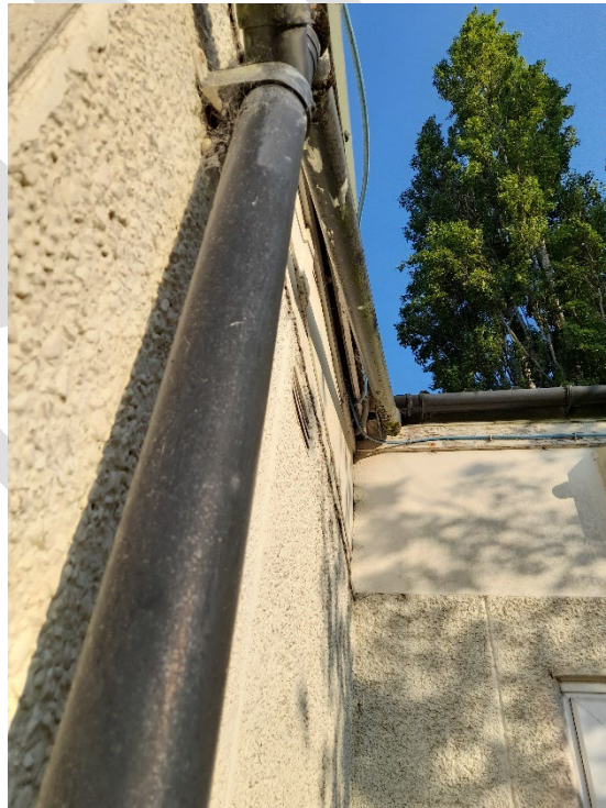
Building 13 – Cavities under fascia on sports pavilion
