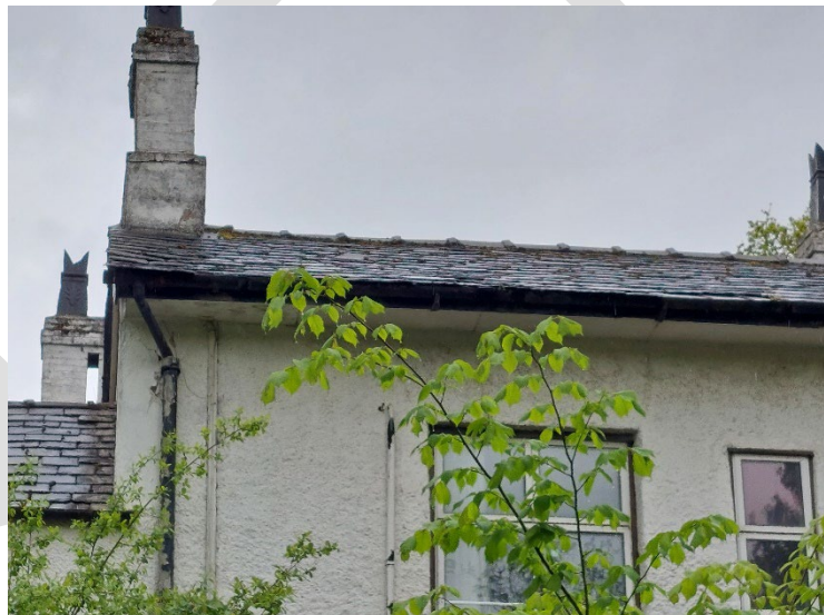
Building 9 – Eastern aspect, showing gaps below ridge tiles on the building extension.
