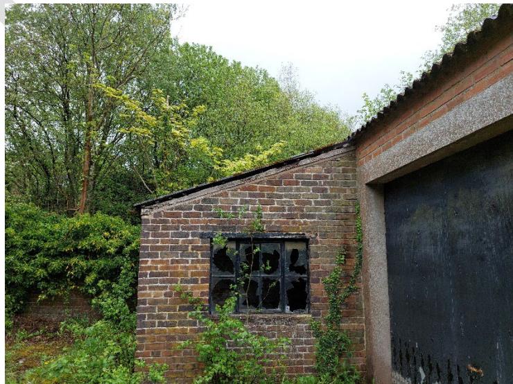
Building 10 – Eastern aspect, showing gaps below the cement sheeting which may lead to the wall plate.
